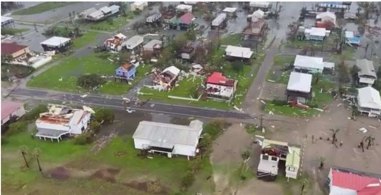
Devastation caused by Hurricane Ida along the Gulf Coast. Photo: US Coast Guard
