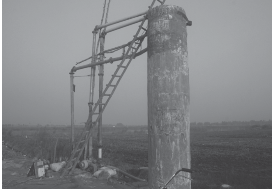
Fig. 3: Water pumps installed on water logged and flooded lands for extraction of water
