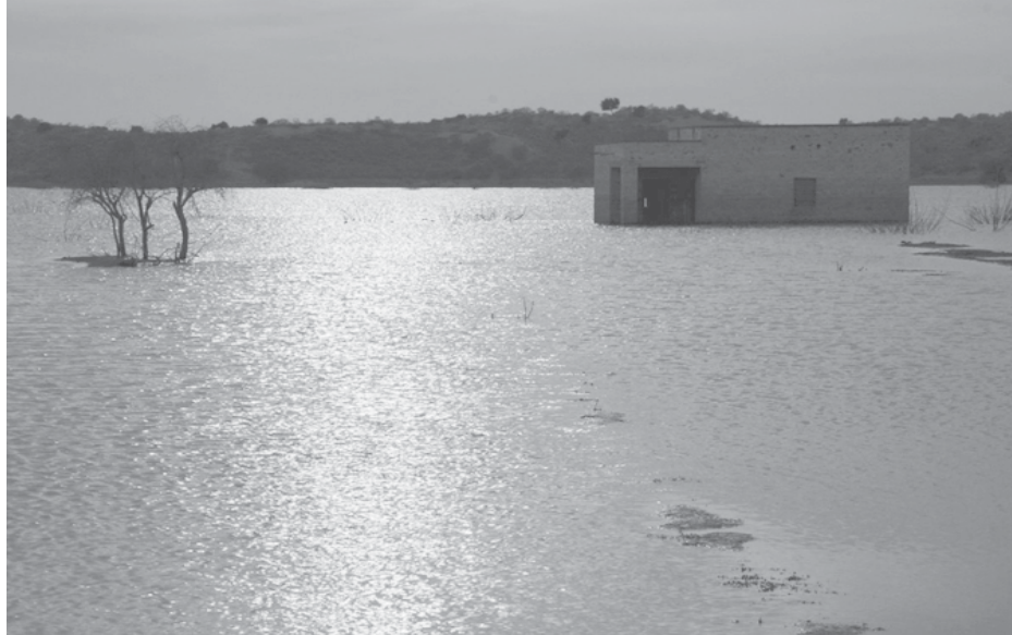
Fig. 2: Flood affected area
