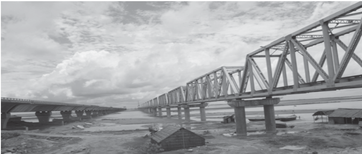
Fig.3: Kosi mega bridge (photograph by Vikas Kumar)
