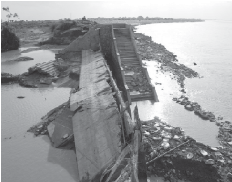
Fig. 5: Damaged weir of a local tank (Source: Authors)
