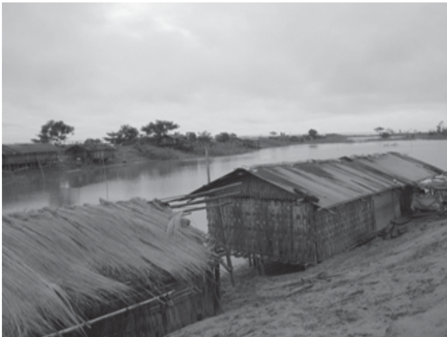
Fig. 3: Houses on the old Sissi-Tekeliphuta Embankment
